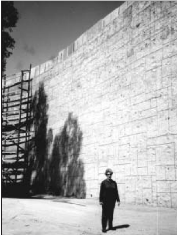
BCA Board Member Sandy Margolis inspects new wall in Benedict Canyon
