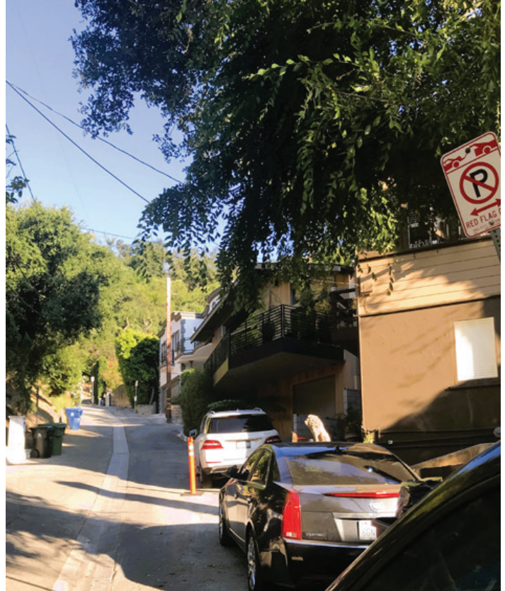
Wanda Park Drive, a sub-standard street, is the proposed entrance for the 8 mega-mansions.
