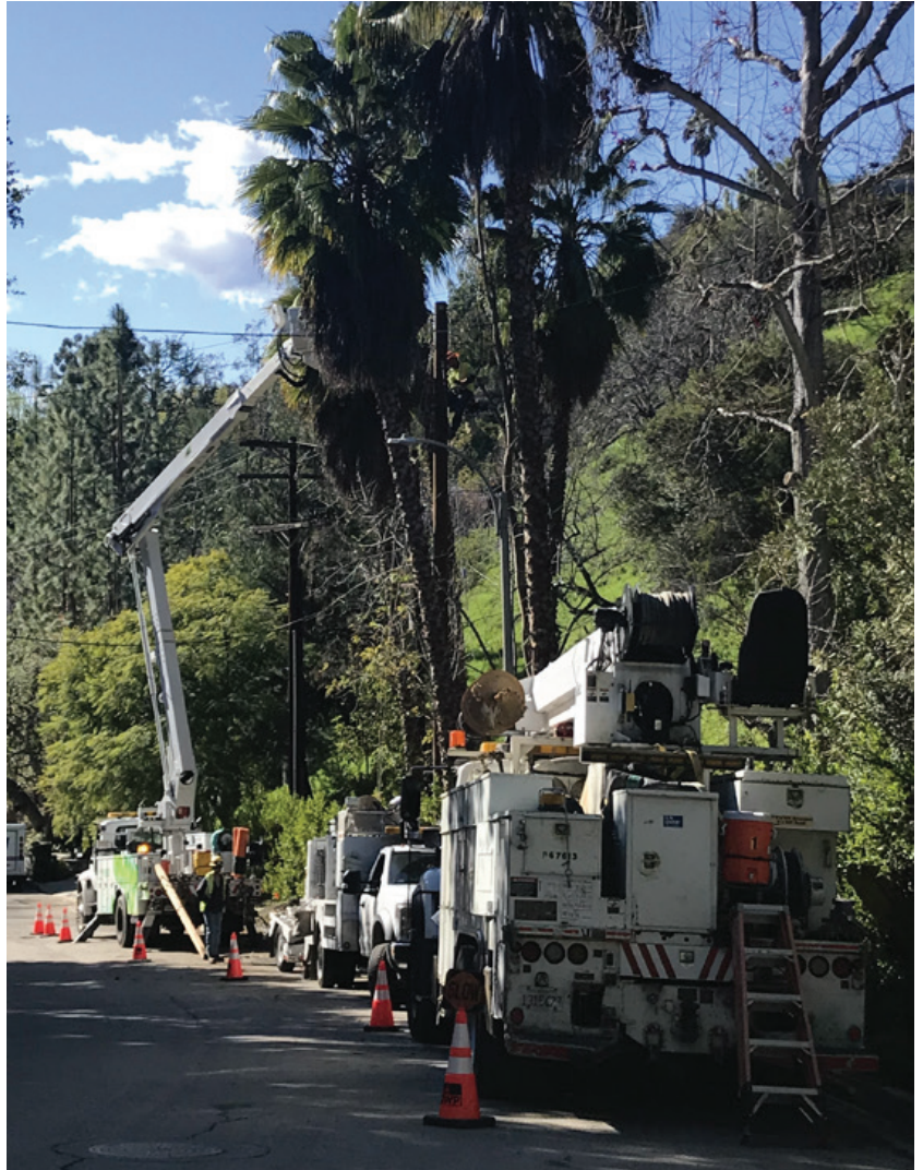
DWP Working on Power Pole
